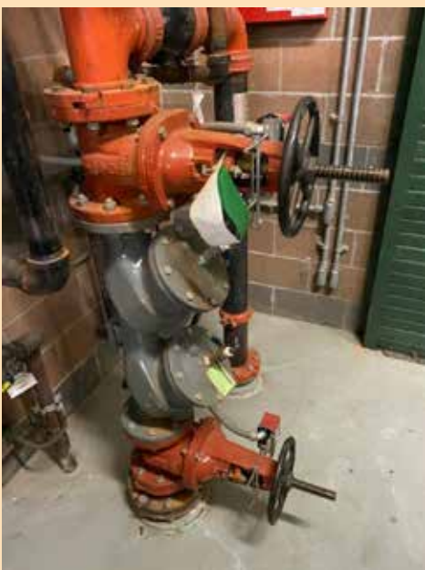
Backflow Assembly Being Tested
